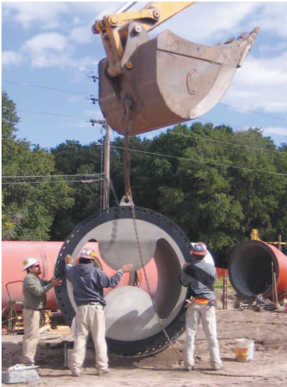
The mixer arrived with pre-applied gasket and pre-drilled flange for easy installation.
